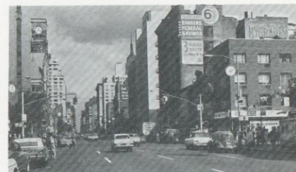
'Village Square'—6th Ave. & 8th St.
