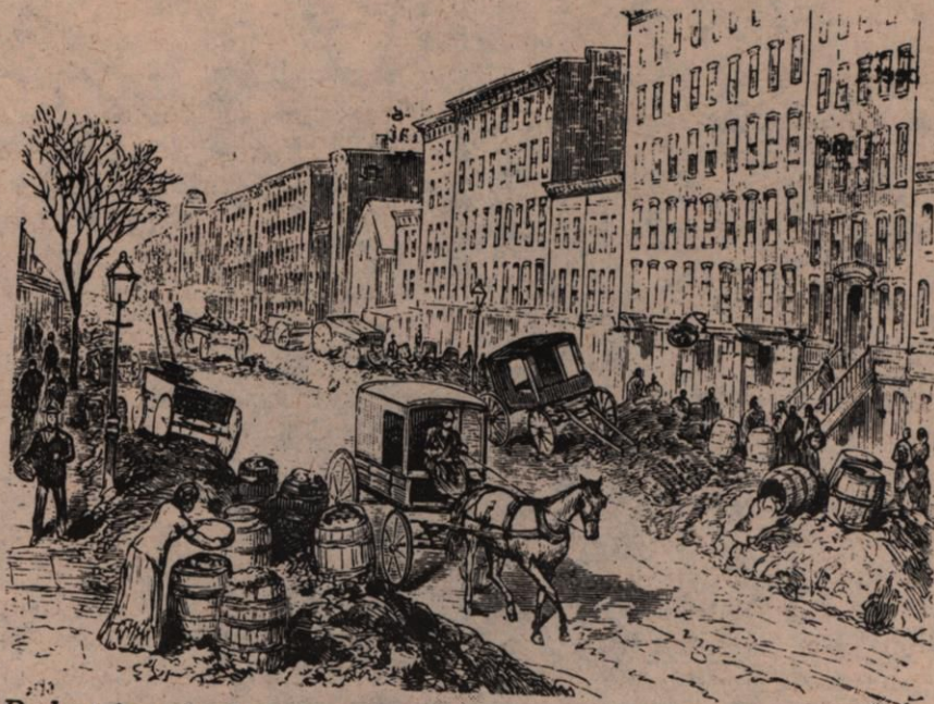
Pedestrians had to step gingerly around sidewalk garbage piles.
