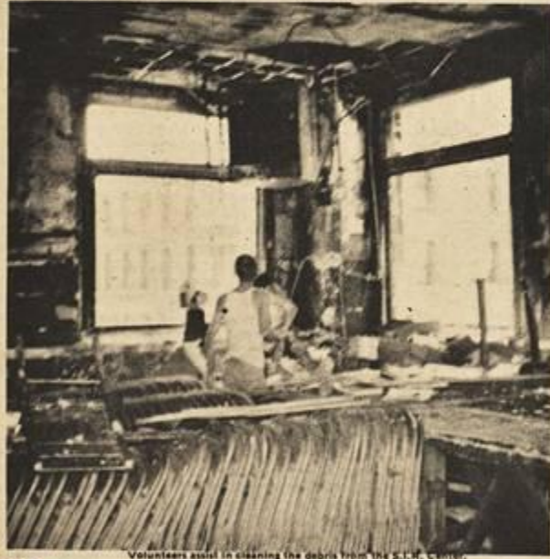
Volunteers assist in cleaning the debris from the S.I.R. Center.
