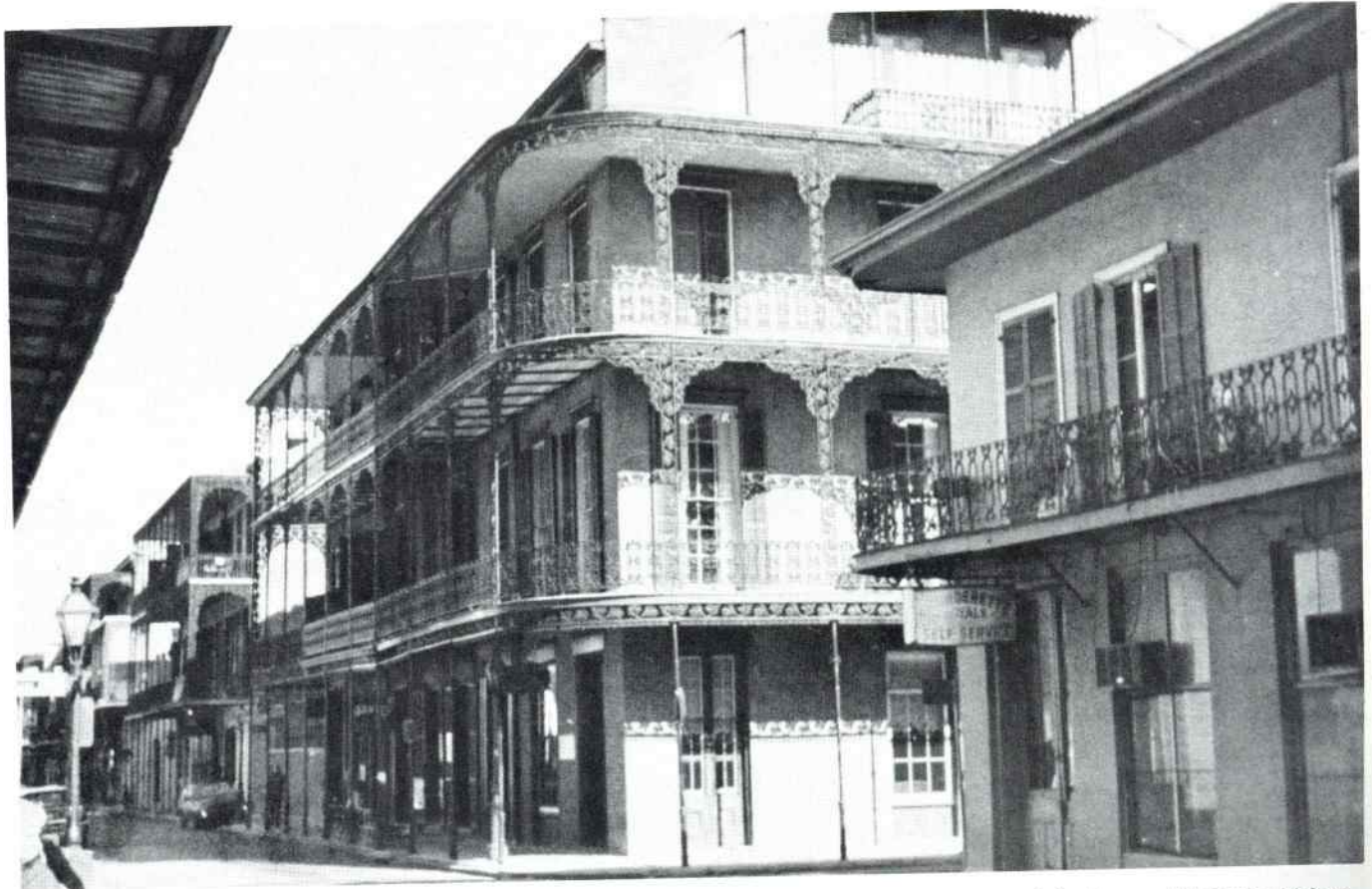
Lace iron work and trellised balconies indicating the French and Spanish influences of architecture add beauty, history and romance in "Vieux Carre" (Old Quarter), more popularly called The French Quarter.
