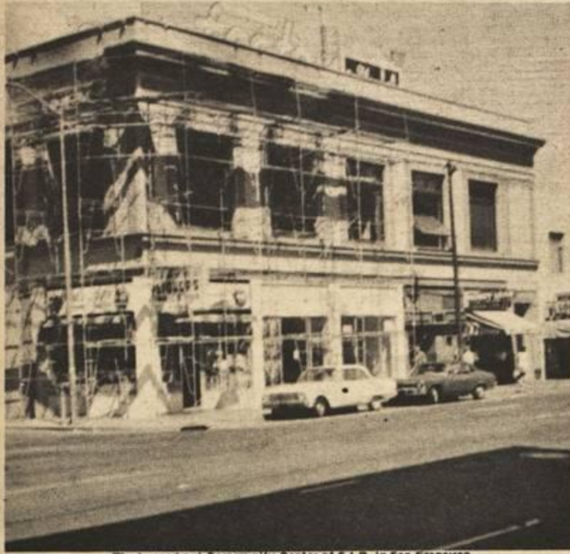
The burned out Community Center of S.I.R. in San Francisco
